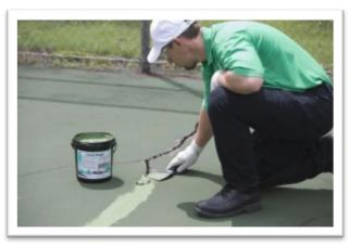
crack and sets up like rubber. Use CrackMagic
