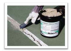
Trowel grade crack fillers, like SportMaster Acrylic Crack Patch, are high in solids, tend to dry quicker, and have more body to fill larger cracks. This product would dry quicker in comparison to a pourable crack sealant. Acrylic Patch Binder is mixed on-site with sand and portland cement, and would also be a great choice for a faster-drying tennis court crack filler.
