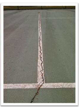
How can this problem be minimized? Lighter <u>tennis court surface colors</u> can minimize the effect so that there is not such a big temperature contrast from the white line to the surface. At minimum, make sure to keep the cracks sealed with an acrylic <u>tennis court crack filler</u>. This will help to maintain the crack and slow down the growth to provide better safety and aesthetics.
